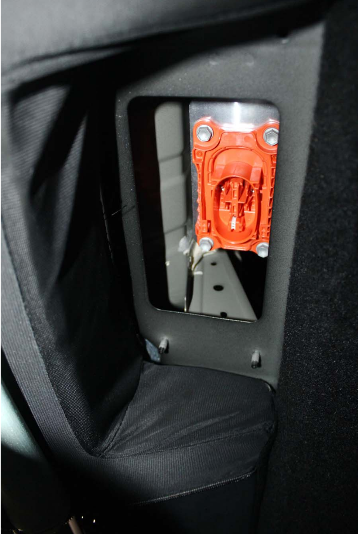
Photo No. 71. Pre-Test Manual Service Disconnect Removed
